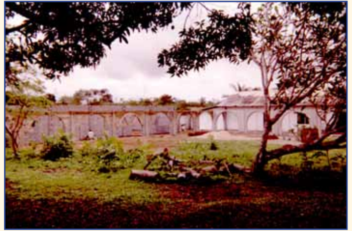
Construction projects in 1998
